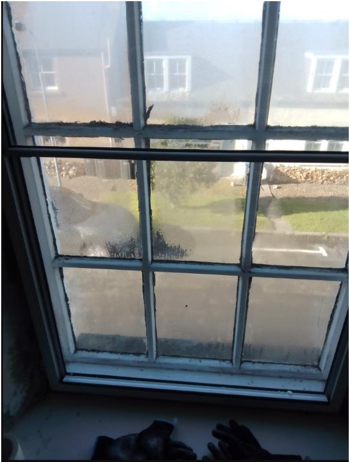
Original Windows and door
